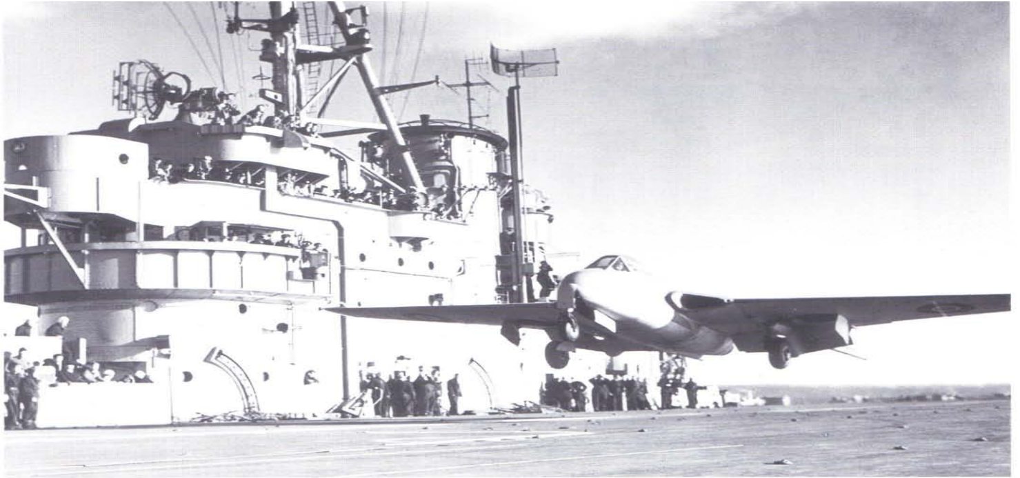
Above: Vampire F.Mk.1LZ551/G landing on HMS Ocean 3 December 1945 by Lt Cdr Eric Brown DSC. It was the first jet landing aboard a carrier. (BAe) Right: The first jet to land on a carrier looking in a sorry state, no engine, no nose-wheel, at RNAS Yeovilton in 1966. It had been made Cat.E (scrap) 13 August 1947 and sold to de Havilland, who passed it on to the Imperial War Museum and has now become one of the exhibits at the FAA Museum. (via Tony Buttler)
